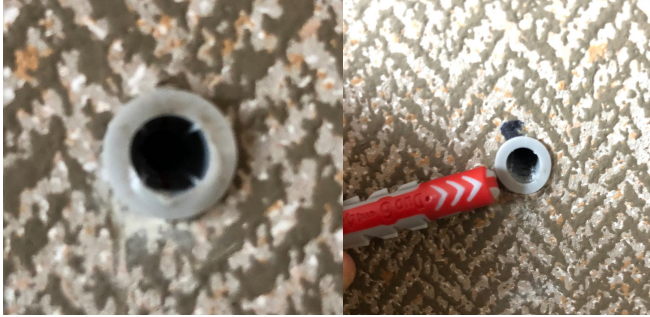
Picture 1. Wall plug in pre-drilled hole
